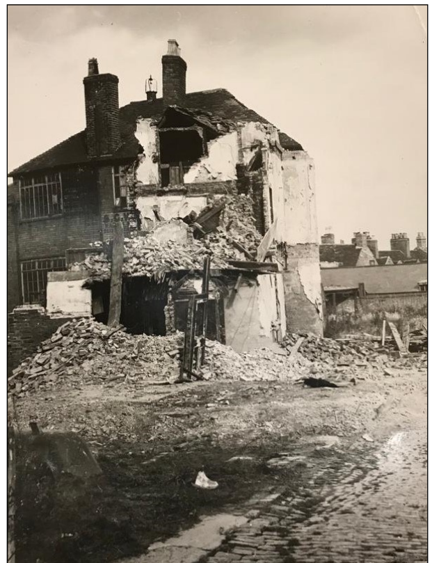
Image depicting the damage caused to 38-39 Bayley Lane.
